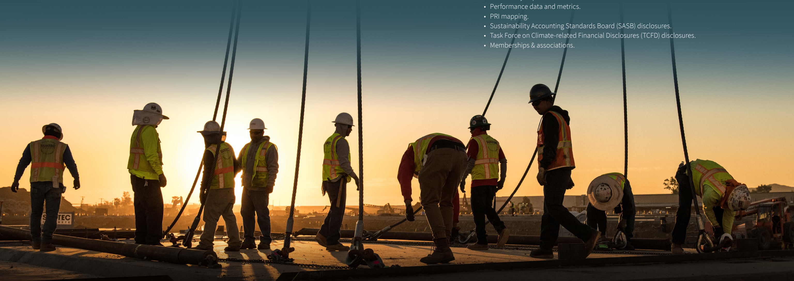
Tilt wall construction at Prologis Park I-17, Phoenix, Arizona.
