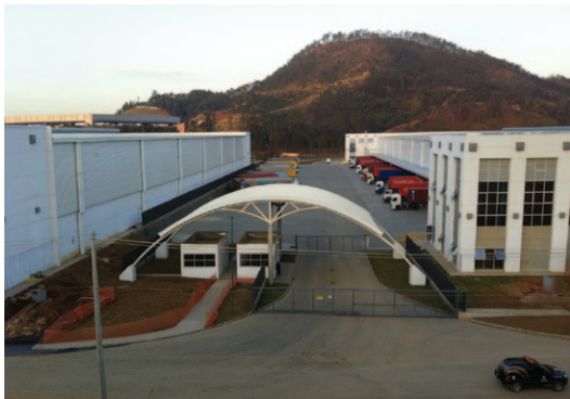
Prologis CCP Cajamar I
