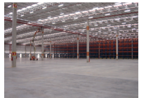
Prologis CCP Cajamar I
