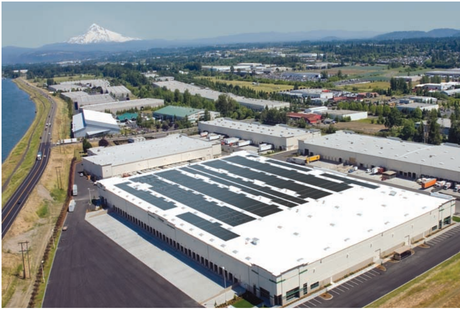
An artist's rendering of a portion of a 1.1 MW solar installation at a distribution center in Portland, Ore. Courtesy of ProLogis.
